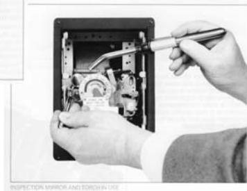
INSPECTOR MIRROR AND TORCH IN USE
