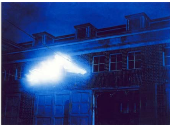
Fig. 8: Short-circuit experiment in the 50 kV power system, Thüringenwerk, 1928
