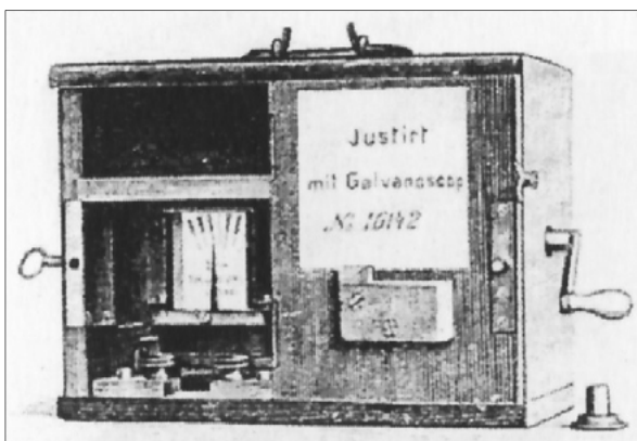
Fig. 1: Insulation tester, S&H, 1886
